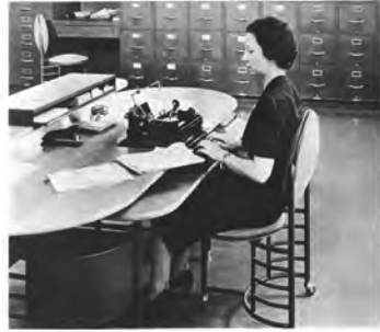
Johnson Wax, administra- tion building, Racine Wisconsin, 1939
