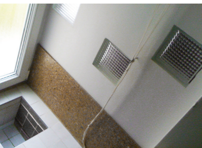
Bathroom, the enclosed flushing system Paris, France (75)
